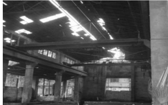
Fig. 10 Damage of envelop enclosure system in single bent frame structure
