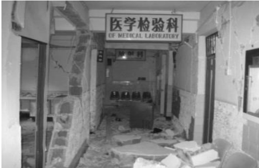
Fig. 5 Collapse of an infilled wall of the second hospital in Dujiangyan City
