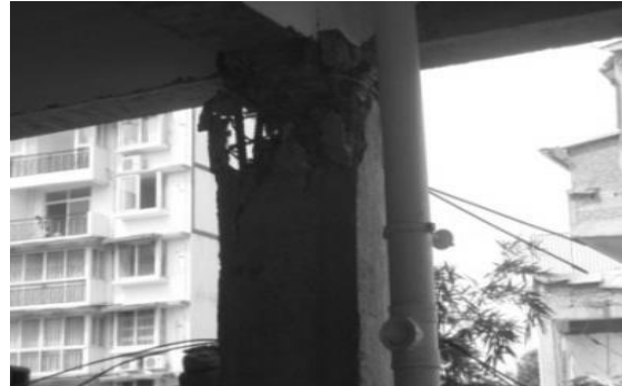
Fig. 6 The lantern-shaped damage of frame column
