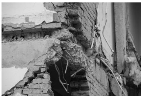
Fig. 3 Structural damage caused by not installing constructional column
