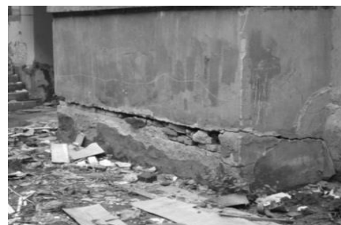
Fig. 4 Masonry structure with cut-through horizontal fracture or crack
