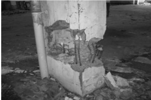
Fig. 9 Damage of bent column in single bent frame structure
