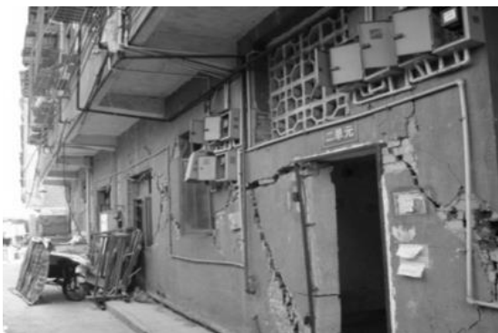
Fig. 7 Damage of masonry structure part in bottom-story hybrid structure
