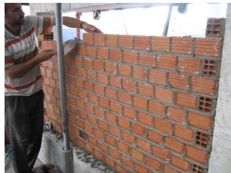
Fig. 7  $\frac{1}{2}$  scaled bricks were used with ordinary mortar
