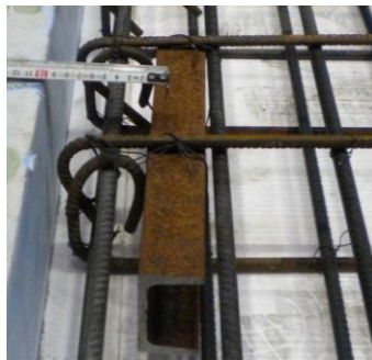
Fig. 9 Detail of specimens CFPU-2 indicating the location of U65 steel element and CFPC-2 indicating the 'gap' arrangement
