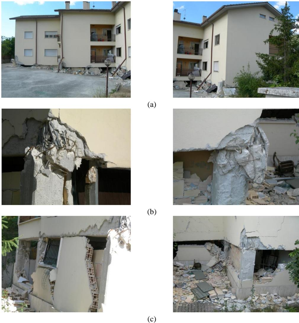
Fig. 4 Damages observed for the studied building: (a) Soft/weak story mechanism, (b) Shear failure in columns and (c) Infills failure
