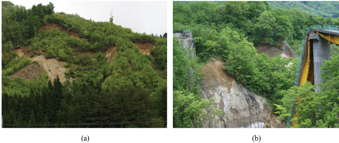
Fig. 1 Earthquake damage: (a) landslide and (b) collapsed bridge
