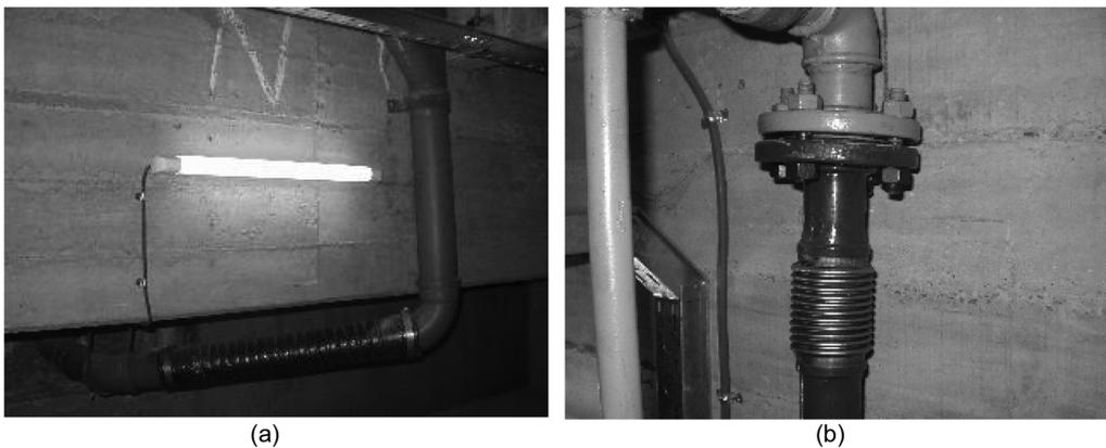
Fig. 2 Flexible joints at isolation level: (a) flexible joint for sewer pipes and (b) flexible joint for gas pipes
