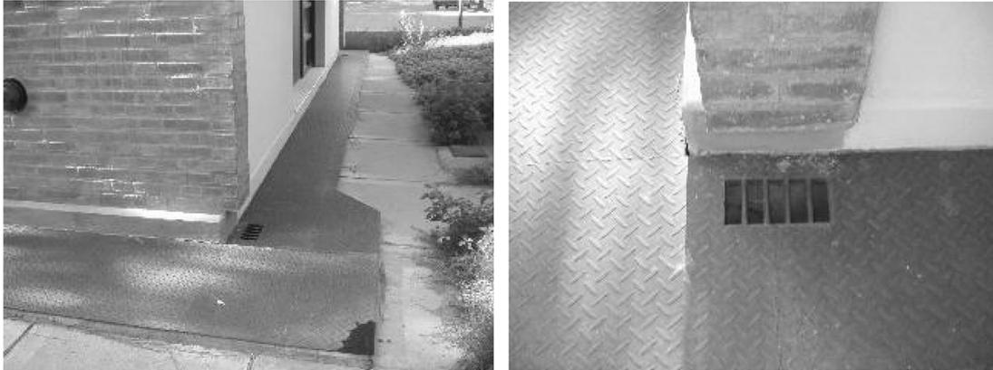
Fig. 3 Structural gaps and steel plate protection
