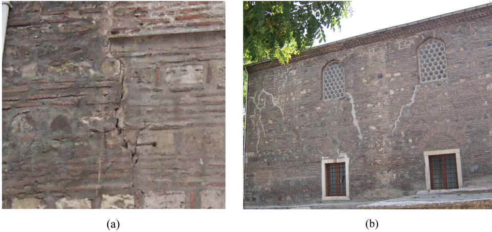
Fig. 2 (a) Vertical wall crack observed after the 1999 earthquakes and (b) repaired cracks in the Imaret mosque
