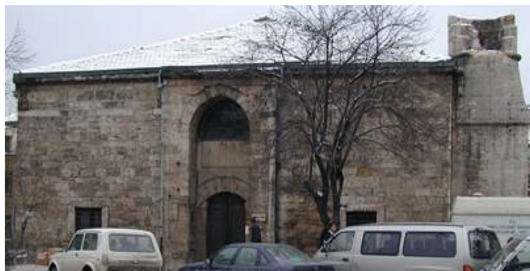
Fig. 5 Entrance of Kadi mosque showing failed minaret
