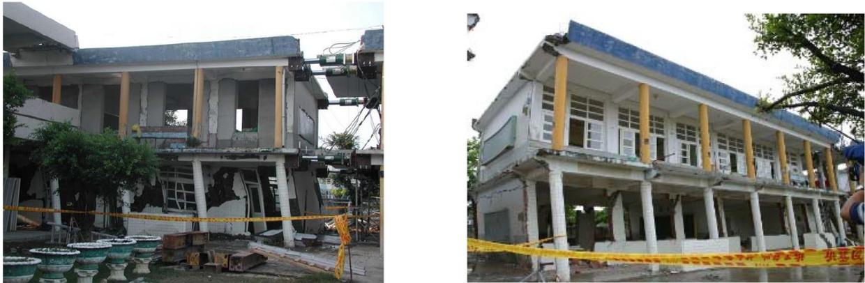
Fig. 15 Pictures of specimen MI (left-hand panel) and specimen BF (right-hand panel) after the field tests
