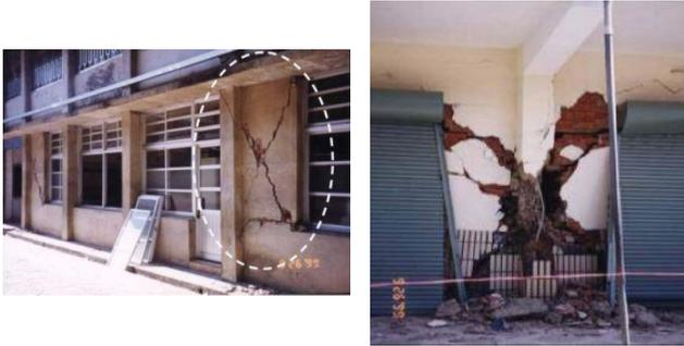
Fig. 1 Photographs of columns that are damaged by infill wall segments
