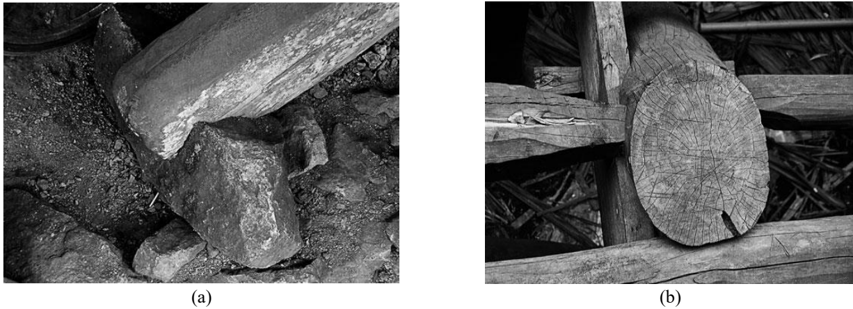
Fig. 9 Connection details (a) between column & stone base, (b) between column & beam
