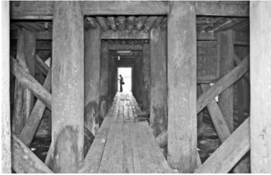
Fig. 5 Dampness on columns and floorboards
