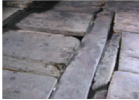
Fig. 5 Dampness on columns and floorboards
