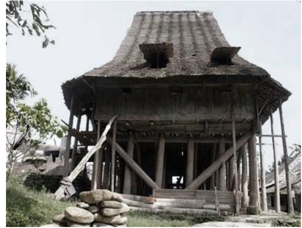
Fig. 1 South Nias typical residential timber house
