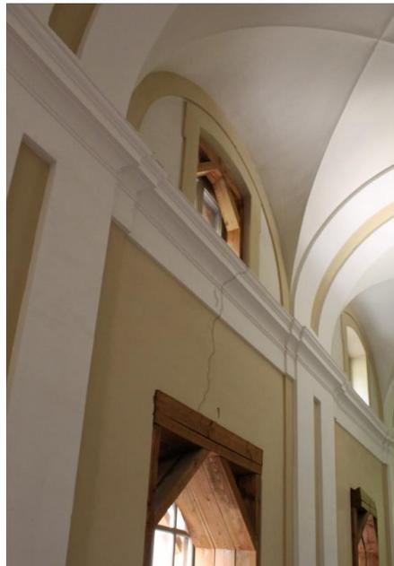
(b) Side of the main corridor characterized by cracks on the masonry architraves and vaults due to the 2009 earthquake
