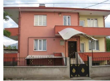
(a) Two story masonry building
