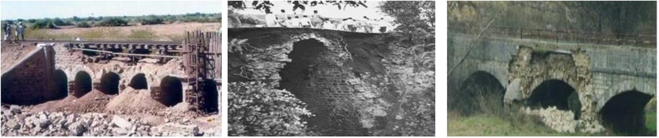
Fig. 4 Some views from spandrel wall failures after earthquakes (Rota (2004))
