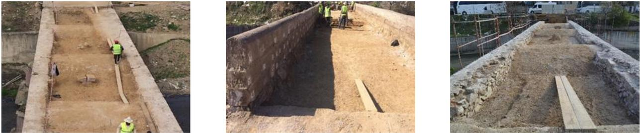
Fig. 2 Views from spandrel walls with soil and mortared rubble backfills
