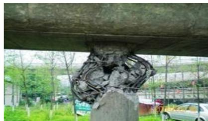
Fig. 1 Shear-bending damage of Hui-Lan curved bridge in 2008 Wenchuan Earthquake
