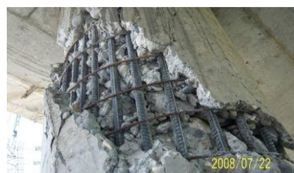
Fig. 2 Collapse damage of Mian-Zhu airport curved bridge in 2008 Wenchuan Earthquake
