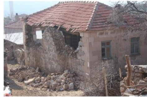
Fig. 7 Use of rubble and cut stone
