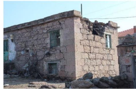
Fig. 8 Use of cut stone around corners and outer parts of the walls
