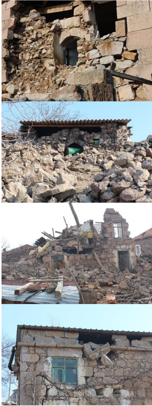
Fig. 10 The effect of door window lintels
