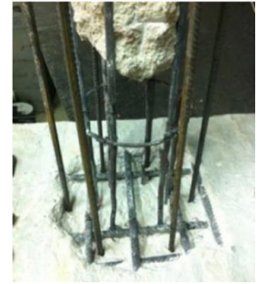
(b) The longitudinal bars of the RC jacket were anchored in the foundation block. The holes were filled with epoxy resin
