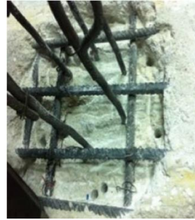
(a) Six \emptyset 12 mm holes were drilled in the foundation
