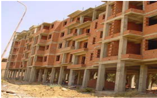
Fig. 1 External panel with masonry infill
