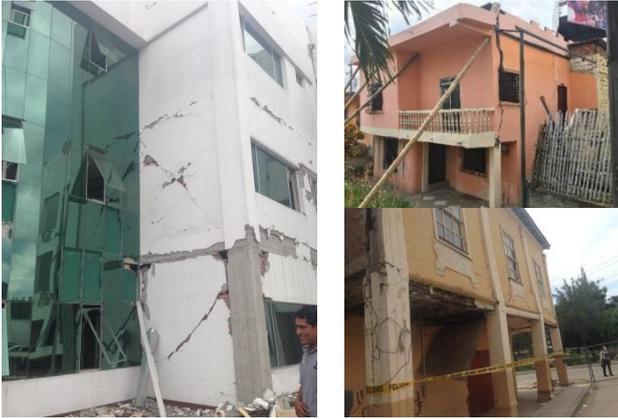
Fig. 1 OoP inter-storey drift failure, Muisne earthquake (Ecuador) (photographs from EERI org 2018)
