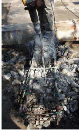
Fig. 7 Extrication of beam reinforcement bars from corroded GLD specimens
