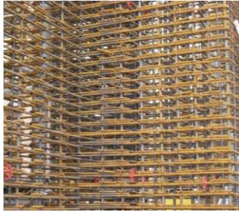
(a) Special details of shear walls
