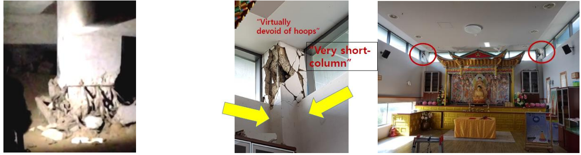
(a) Failure of column at the base of structure (KBS)
