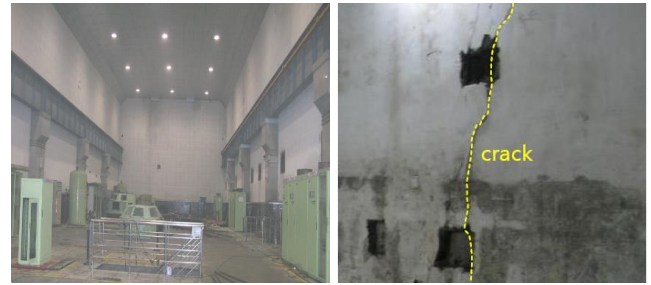
(a) Underground powerhouse (b) Crack in the traffic tunnel
