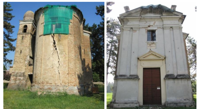
(a) Overturning mechanism (b) in-plane failure of the main façade
