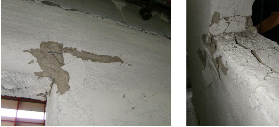
Fig. 10 Damage at the corners of the openings (i.e., door and window)
