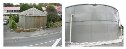
Fig. 1 Foundation sliding (right) and wall damaged due to sloshing motion (left) in Darfield earthquake (2010) (Courtesy of Timbertanks)
