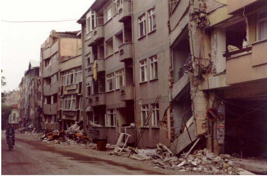
Fig. 5 Soft storey effect in buildings during Marmara earthquake, Turkey (1999)
