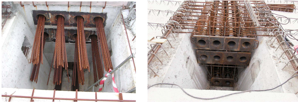
Fig. 8 Anchorage devices of tendons before post-tensioning
