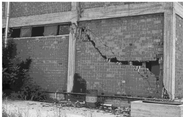
a) short column damage
