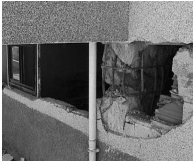
Fig. 3 Shear failure at short column (Erdik et al. 2003)
