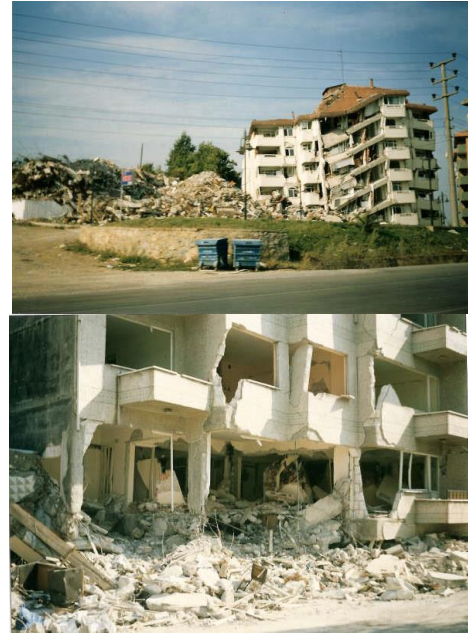
Fig. 2 Typical damages in R/C buildings after 1999 Marmara earthquakes in Turkey
