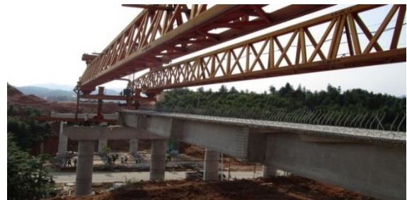
Fig. 1 Bridge construction using PC T shaped bridge girder (Peoplerail.com 2017)
