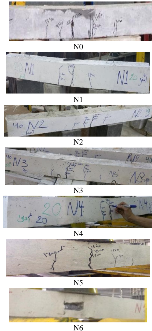
Fig. 5 Crack pattern for the tested beams
