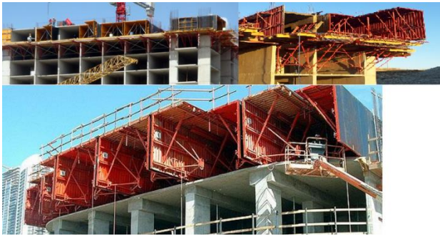
Fig. 2 An RC structure constructed by TCF
