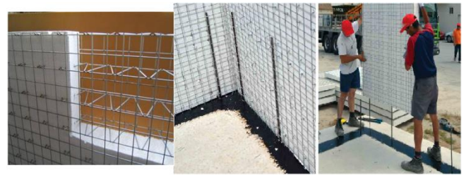
Fig. 3 An RC structure constructed by lightweight prefabricated 3D Panel
