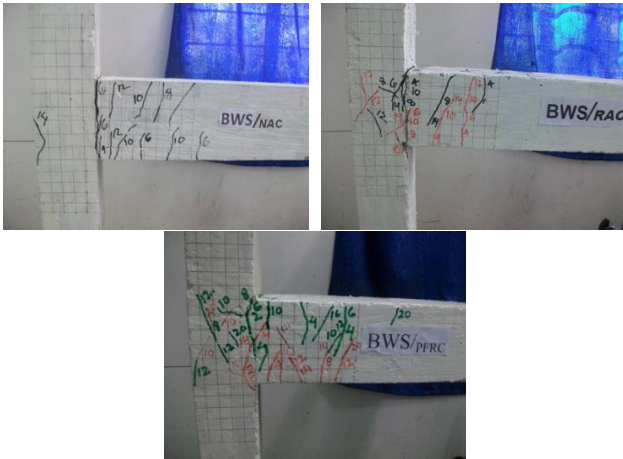
Fig. 9 Failure modes of BWS specimens
