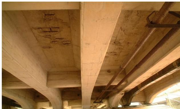
Photo 1 Deterioration of the KT-Bridge
