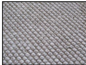
Fig. 3 Homogeneously roughened concrete surface
