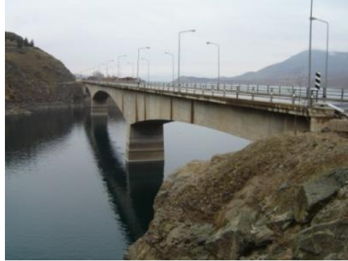
Fig. 6 A view of Komurhan Bridge
