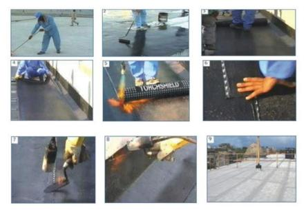
Fig. 1 Waterproofing for roofs with bitumen felt
