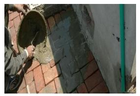
Fig. 7 Smoothing of cement grouting
