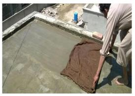
Fig. 6 Grouting of joints
