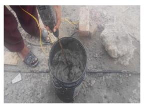
Fig. 2 Mixing of PPPMS slurry with water
