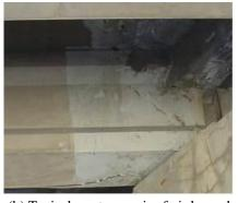
(a) End damage of girder(b) Typical mortar repair of girder endFig. 12 End region damage and mortar repair of concrete bridge girder
