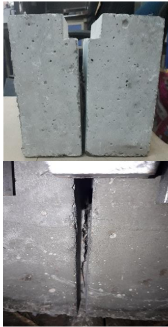
Fig. 6 Failure pattern of specimens with guide notch
