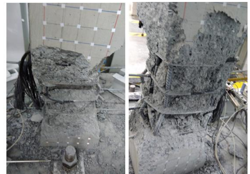
Fig. 10 Various damage photos for S453508
