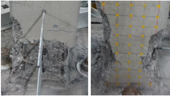
Fig. 8 Various damage photos for S452008
