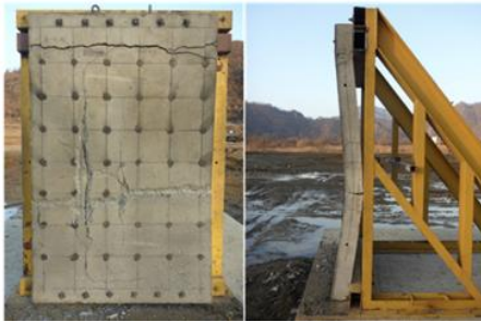
(b) Hazardous failure
