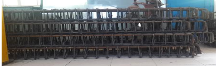
Fig. 4 Pre-fabricated reinforcement cages
