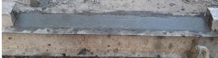
(b) Casting of RC beams
