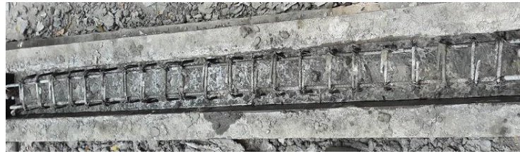
(a) Steel molds for RC beam with reinforcement
