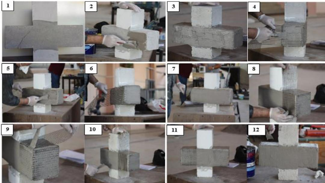
Fig. 3 Configuration steps of the bonding surface and applying the Basalt Fiber Mesh with epoxy to the damaged corbel from 1 to 12 steps
