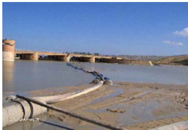
Fig. 3 Dredging operation through the outlet pipe
