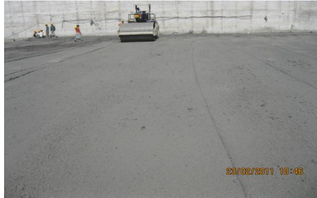
Fig. 6 RCC surface after compaction at Middle Vaitarna
