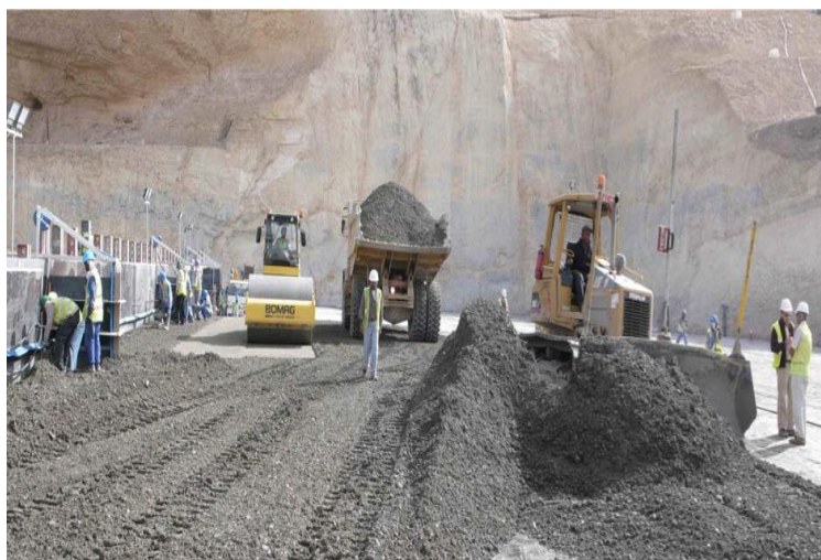
Fig. 5 RCC construction- dumping, spreading and compaction
