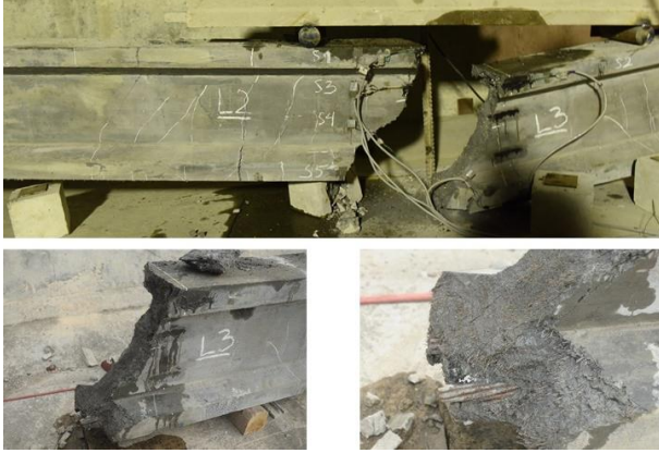
Fig. 12 The rupture failure mode of I-girder
