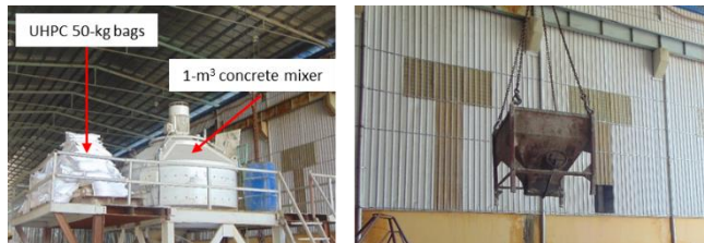
Fig. 1 The industrial concrete mixer and the facilities of the local precast plant
