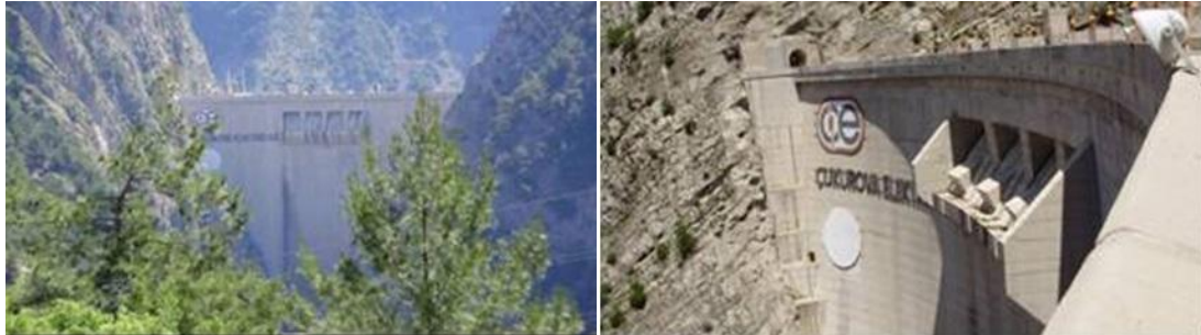
Fig. 1 Some photographs of berke arch dam
