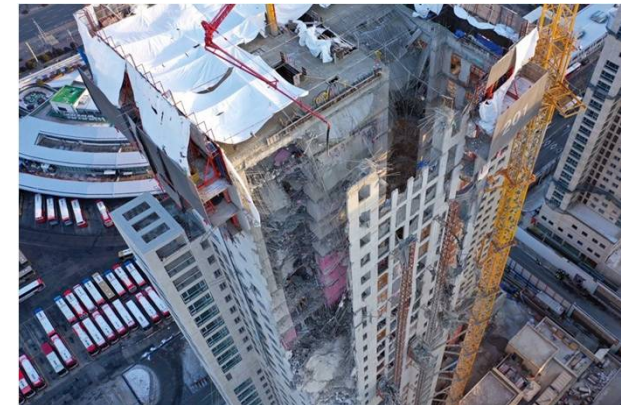
Gwang-ju Apartment Collapse (2022)
