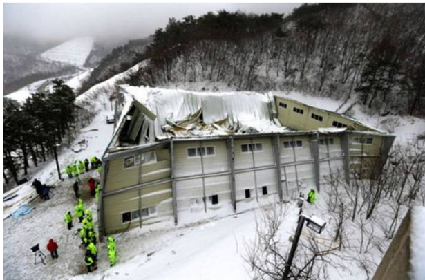
Gyeongju Mauna Resort Collapse (2014)
