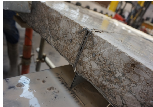
Fig. 3 Embedded edge trims shown after transverse cutting
